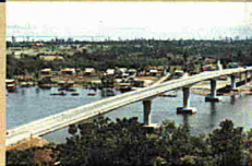
North Westerly view of the Bridge Sulaman Coastal Road
