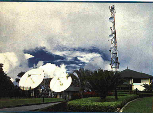
The MEASAT Satellite Control Centre (MSCC) in Pulau Langkawi.
